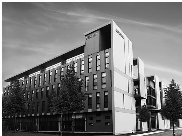
“诺雅克”松江工业园一角
